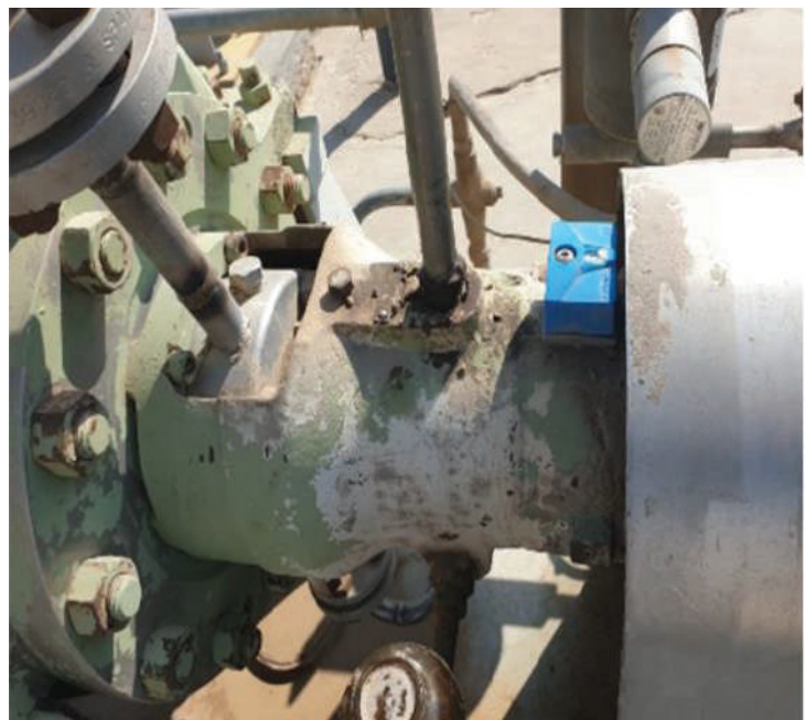
Field implementation of the wireless monitoring device
